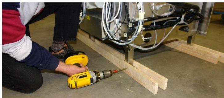
All the screws and bolts of the packing are now removed.
