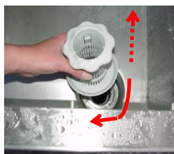
Remove the outlet screen.
