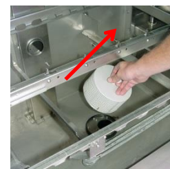
Remove the pump suction sieve.
