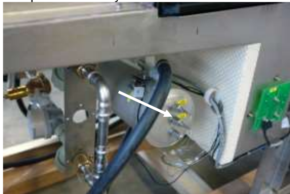
Temperature safety limit switch on the flow heater:
